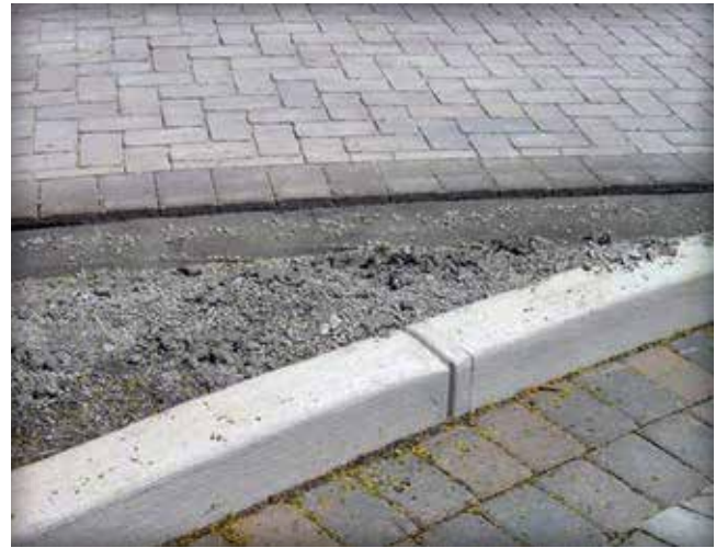
Figure 20. A PICP walk with a troweled concrete toe sits next to a driveway with a formed and cast-in-place concrete curb. Concrete toes should only be used for pedestrian applications.
