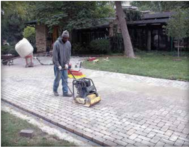
Figure 19. Edge restraint is spiked into the dense-graded base berms so it can hold the pavers in place during compaction and service.
