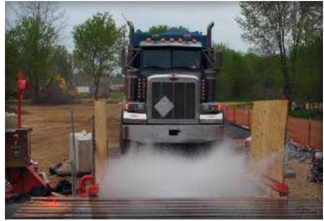
Figure 11. Larger PICP projects may require tire washing equipment for trucks to keep mud from contaminating PICP aggregates.
