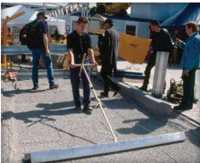
Figure 25. Manually screeding the No. 8 stone setting bed.
